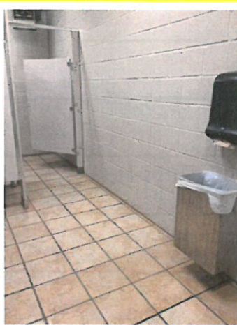
Remove trash, sweep and mop restrooms.
